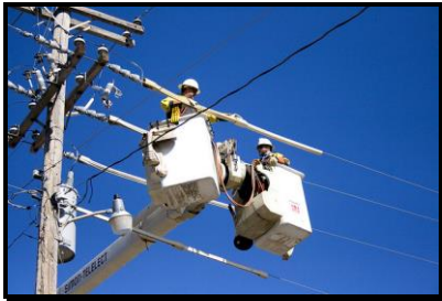
Linemen at Work
