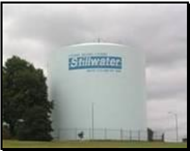
Water Storage Tower
