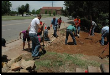
Construction of Rain Garden
